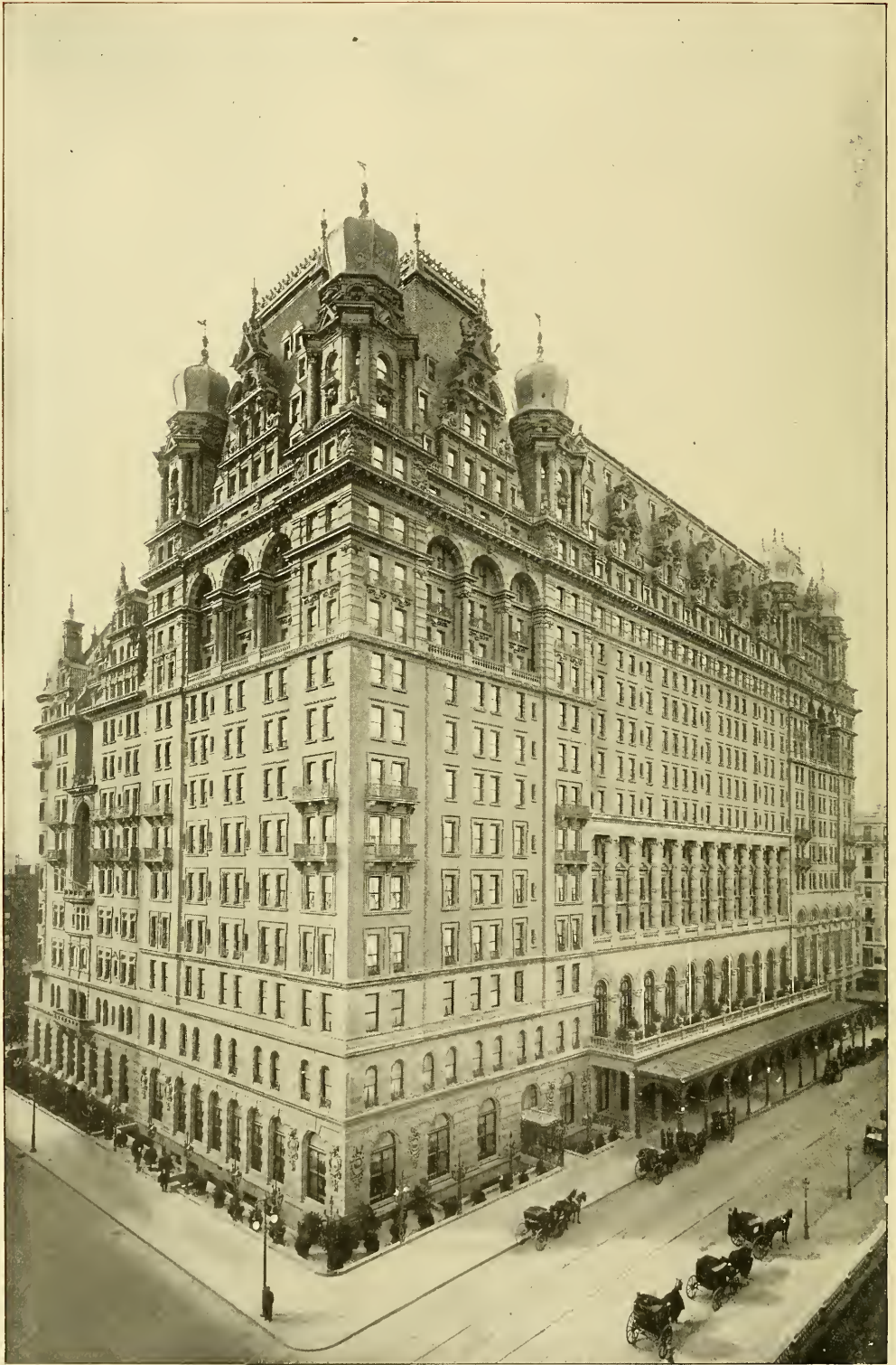
Waldorf-Astoria Hotel, New York. 2257 H.P. Babcock & Wilcox Boilers.
